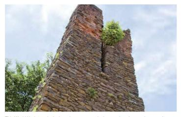
This World Heritage site in the culture category is the remains of a reverberatory furnace built in 1856 by the Hagi Domain that aimed at casting Western-type iron cannons. The reverberatory furnace is a metal smelting furnace necessary for casting cannons. Currently, the 10.5 m high chimney is the only part that remains.
