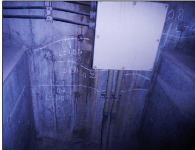
ひびわれ [w=1.1mm L=0.5m] [w=0.25mm L=0.85m] [w=0.2mm L=1.0m]
