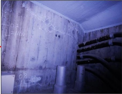
ひびわれ [w=1.1mm L=0.6m] [w=0.25mm L=1.5m] [w=0.8mm L=1.2m]
