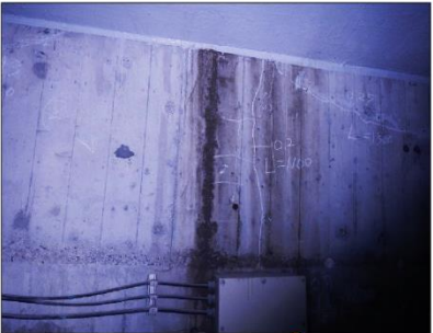
ひびわれ [w=0.8mm L=0.8m] [w=0.4mm L=0.6m] [w=0.1mm] [w=0.4mm L=1.0m]
