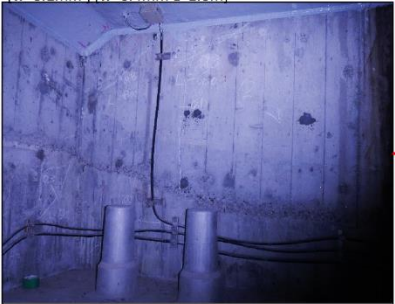
ひびわれ [w=1.1mm L=0.5m] [w=0.25mm L=0.85m] [w=0.2mm L=1.0m]
